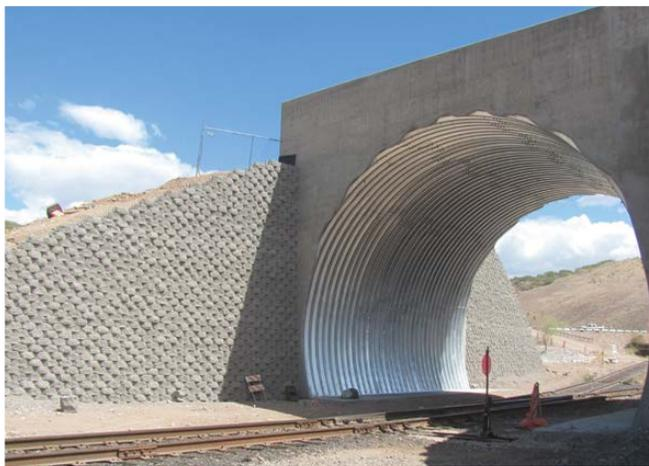
BridgeCor® structures enhance the established performance of 6" x 2" MULTI-PLATE by offering 9 times the stiffness and 3 times the strength
