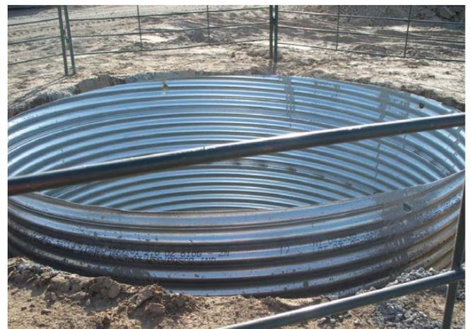
CMP is used as a deep foundation form at the base of the windmill
