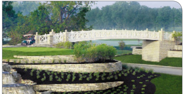
Bridgewater Club – custom-designed pedestrian truss complements the club architecture, with deck lighting and ornamental treatment on the railing posts
