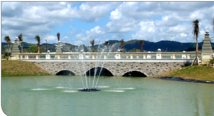
Los Lagos at Palmas del Mar – functional and aesthetic multi-span golf cart bridge treated with stonework on the facade
