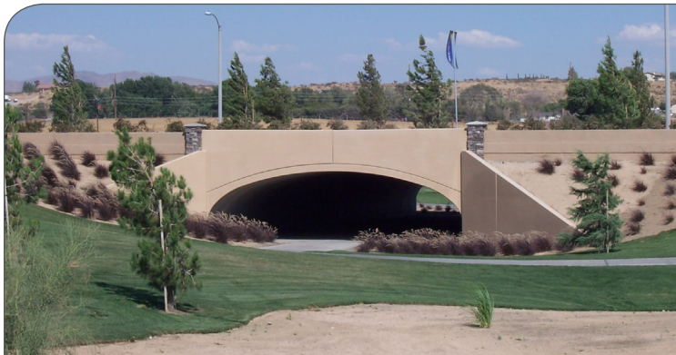
Jess Ranch Golf Course – single-span underpass serves as grade separation for golf cart path and carries residential roadway traffic
