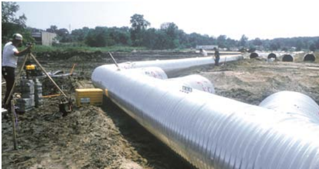
A CORLIX storm sewer system with prefabricated stubs eliminates the need for forming concrete junction boxes.
