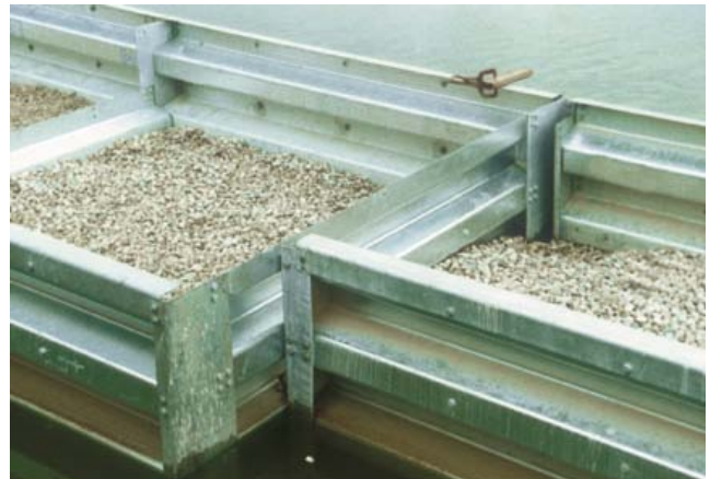
Bins with 1/4" and larger granular fill material.
