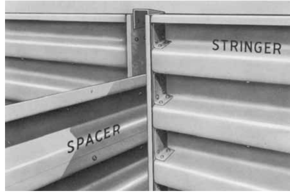
View from back of bin to inside of face. Note how the stringers and spacers are securely joined to the vertical connectors to make a completely closed bin.
