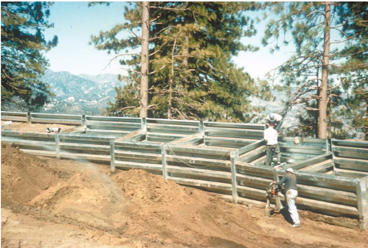
Tamping each layer of backfill to optimum density produces the maximum design strength of the Bin-Wall.
