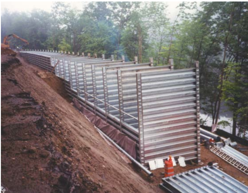
Height-to-depth ratios for Bin-Wall typically require less excavation than cantilever concrete retaining walls or modular block retaining walls.
