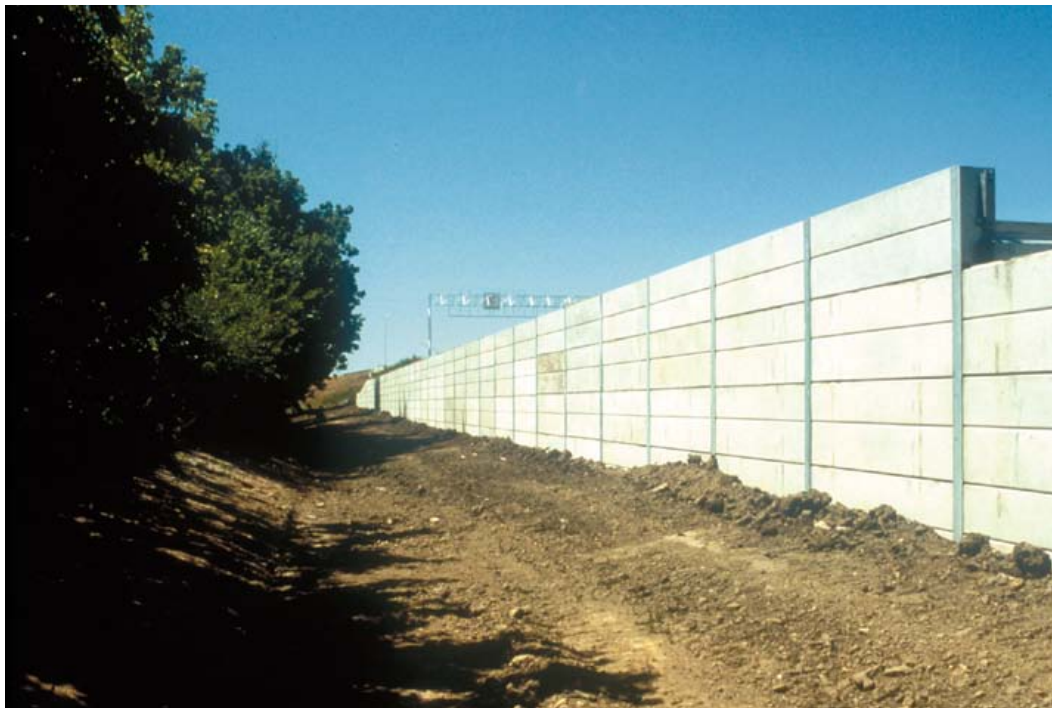
Contech Bin-Wall faced with reinforced concrete panels.
