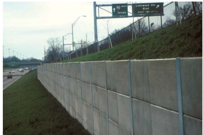
Concrete-faced bin-wall along interstate highway.
