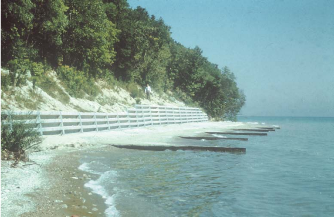
Milwaukee, Wisconsin—installed in 1948
