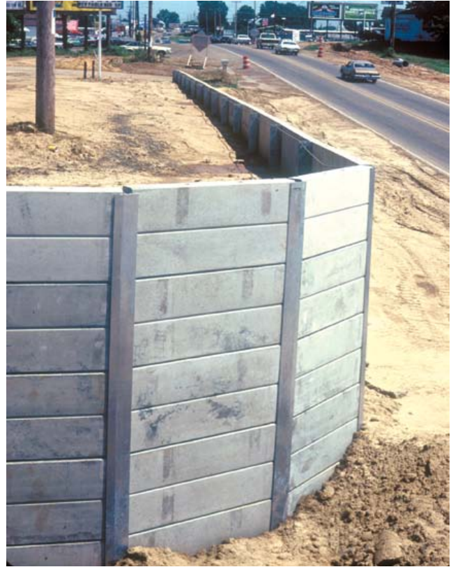
Bin-Wall system allows angle changes.
