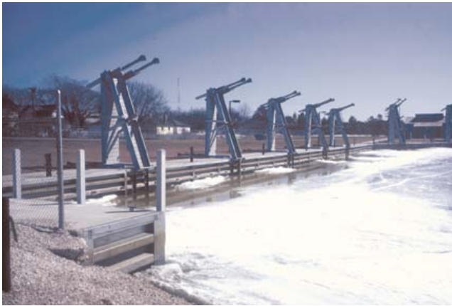
Bin-Wall supports folding slips at Manistique, Michigan Marina
