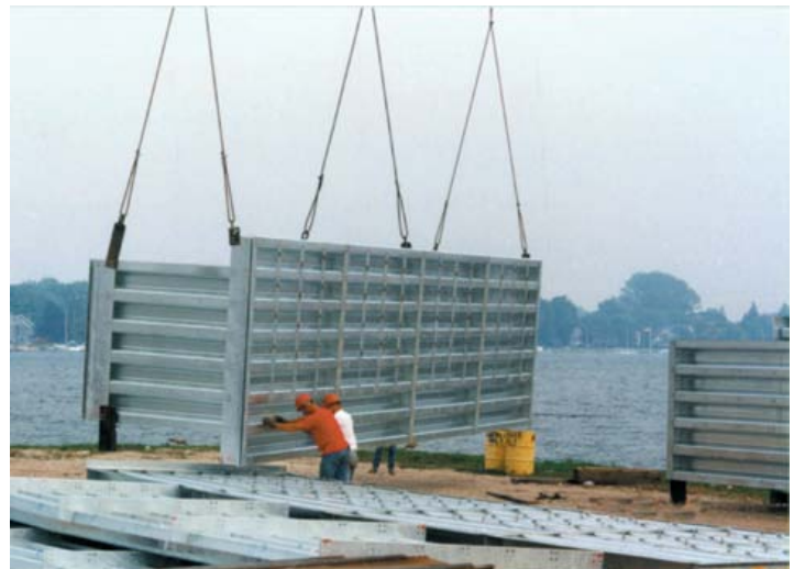
Crane lowers a preassembled bin section into place.
