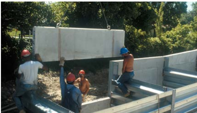
Concrete panels easily slide into place.
