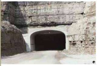
Sugar Creek Mine (MO) — protection from falling rocks (CON/SPAN)
