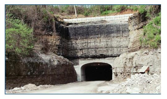
Due to the concerns of falling rock at one of their limestone facilities, LaFarge North America (LNA) needed to secure the mine entrance from debris as soon as possible.
