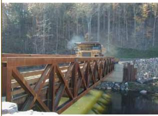
**Baker Industrial Bridge (WV)** — supports heavy construction equipment (Vehicular Truss Bridge)
