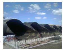
One particular drainage crossing was analyzed as a major bridge crossing, so Marston Environmental contacted Contech to discuss the available options. After considering a BEBO<sup>®</sup> Concrete Arch structure, it was decided that a 5-Barrel MULTI-PLATE pipe-arch structure was needed in order to pass the required flows for the specific location.
