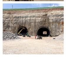
As a solution, four 41'-6.5" x 29'-8" BridgeCor® 63S Single Radius Arches, 30 linear feet in length, were installed in the tunnels as outfall protection canopies. The structures had a hot-dipped galvanized finish with the portion within the tunnels shotcreted to seal any gaps.
