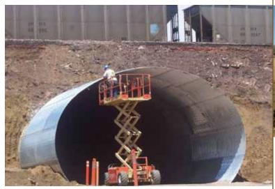
**Jacob's Ranch Mine (WY)** — extends mine entrance to accommodate third rail line (SUPER-SPAN)
