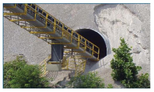
The Rogers Group needed a solution that could accommodate a conveyor system for a rock quarry in Louisville, Kentucky. Contech provided a 14' diameter MULTI-PLATE structure designed with external ring stiffeners/ring beams, and 96 feet of 48" corrugated metal pipe utilized for the escape tunnel. The height of the pile will not exceed 60'.
