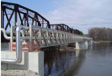
**Long Span Solutions** — single truss pieces can be combined to span large areas or waterways
