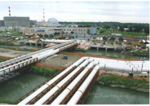
**Multiple Structures** — support 72" diameter pipes carrying extreme temperature liquids at a nuclear facility
