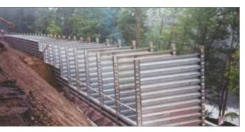
Application: Gravity-Type Retaining Walls for Mining Use
