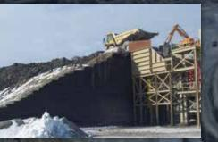
WIRE FACED WALLS » assembled structures
