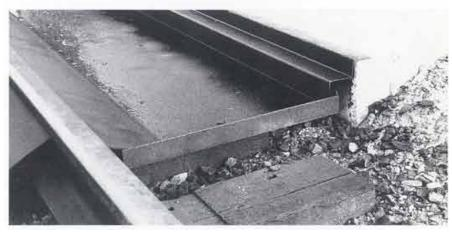
On this installation, concrete platforms were poured with a nosing angle on the edge. A zee flashing angle is welded to the angle, protecting against oil leaksage.
