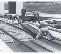
On this installation, concrete platforms were poured with a nosing angle on the edge. A zee flashing angle is welded to the angle, protecting against oil leaksage.
