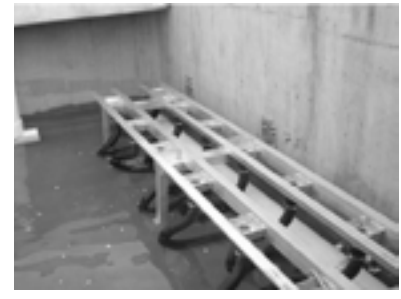
Figure 3. Cartridge support rack Down (Operation Position)
