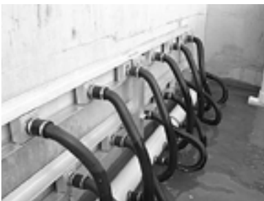
Figure 4. Cartridge support rack Up (Maintenance position)
