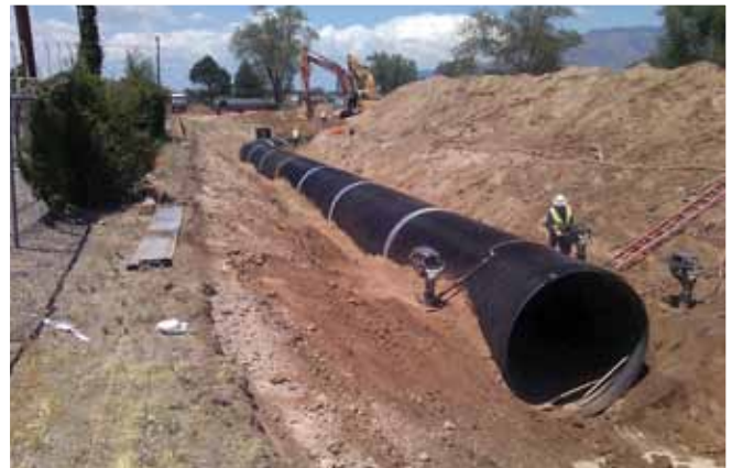
96" diameter DuroMaxx SRPE Pipe installed in New Mexico.
