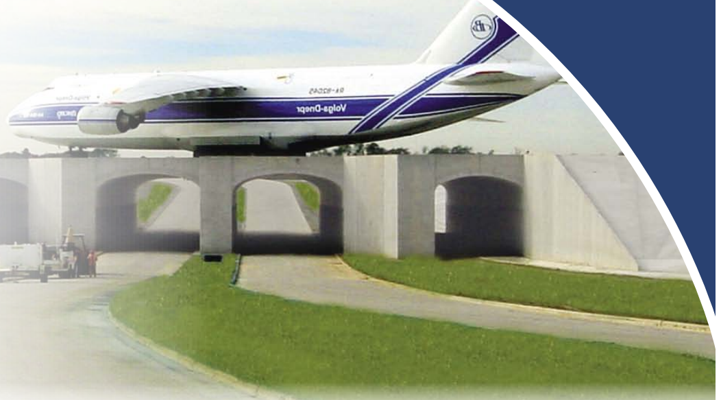
Taxiway Bridge – runway expansion at Houston Intercontinental Airport supports 1.6 million pound payload
