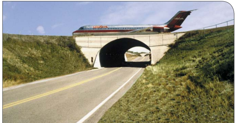
Taxiway Overpass – supports special aircraft design loading at the Port Columbus Airport (SUPER-SPAN™)
