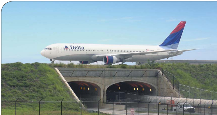
Runway Extension – design supports aircraft loading on extended taxiway at the Hartsfield Atlanta Airport
