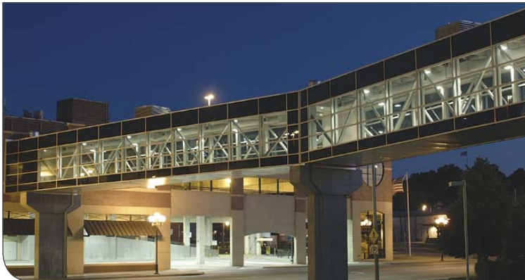
Pedestrian Access – truss structures can be used as walkways to connect facilities
