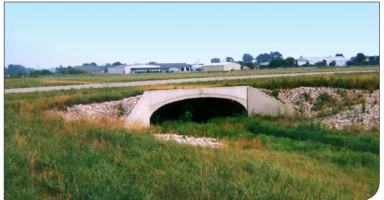
Stream Crossing – allows continuation of runway over a stream cutting through the Greenwood Airport in Indiana
