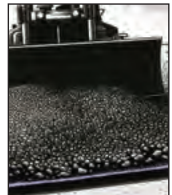
Geotex® heavyweight nonwoven geotextiles allow the construction of landfill drainage layers without fear of liner damage.
