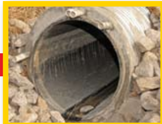
Different length PVC pipes that will deliver the grout flow are installed, and both ends of the pipe are sealed.
