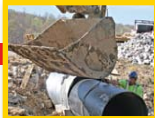
The first piece of Snap-Tite® HDPE is lowered into position and inserted into the host pipe.
