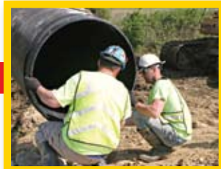
A gasket is installed on the next piece of pipe, assuring a watertight seal when connected, meeting ASTM D3212 requirements.
