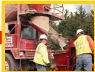
Workers prepare the low density cellular grout that will be pumped into the pipe.
