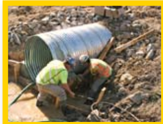
The same culvert, excavated and prepared for Snap-Tite® rehab. Since the pipe was so deteriorated, this project required the installation of a corrugated metal sleeve to accept the new pipe. A concrete footer was also poured.
