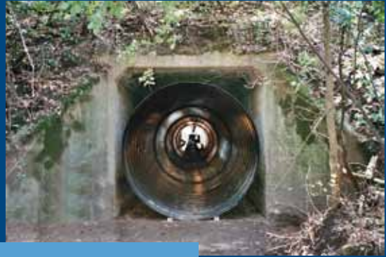
Corrugated Steel Pipe was used to repair a failing reinforced concrete box under a height of cover of 91 feet. Grout plugs were furnished to facilitate concrete grout placement between the new corrugated steel pipe and the existing concrete box.
