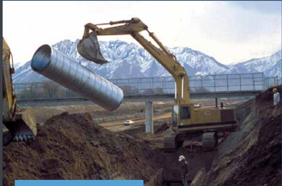
Long lightweight sections make corrugated steel pipe easy to install.
