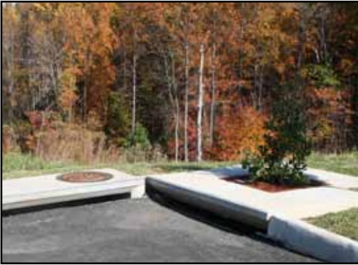
1. Inspection of Filterra and surrounding area
