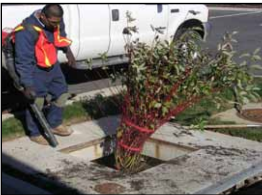
5. Clean area around Filterra
