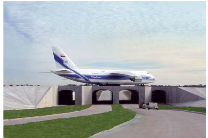
Airport Runway — Precast arch units provide a perfect solution to airplane runway extensions
