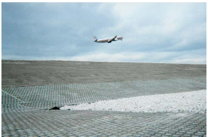
ArmorFlex® closed-cell blocks are ideal for retention ponds as they prohibit vegetation and discourage wildlife and waterfowl from gathering to increase safety for runways and taxiways.
