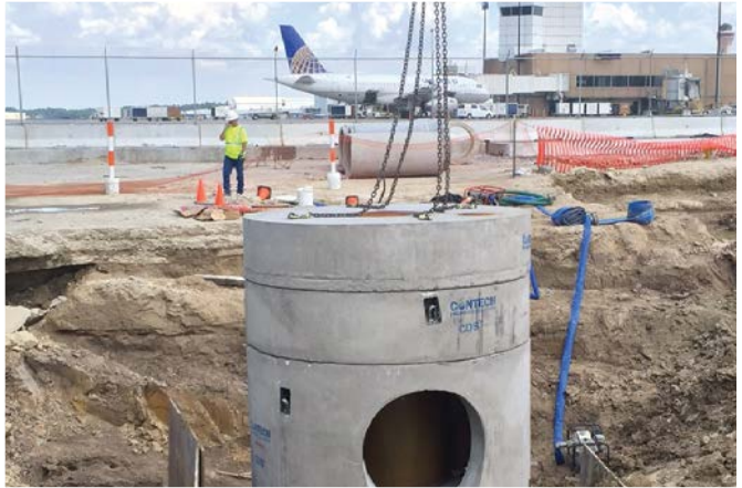
CDS® can be designed to withstand aircraft loading while the flexible configurations allow for efficient handling and treatment of stormwater runoff. George Bush Intercontinental Airport - Texas
