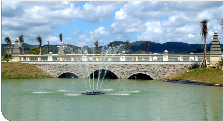
Los Lagos at Palmas del Mar – functional and aesthetic multi-span golf cart bridge treated with stonework on the facade
