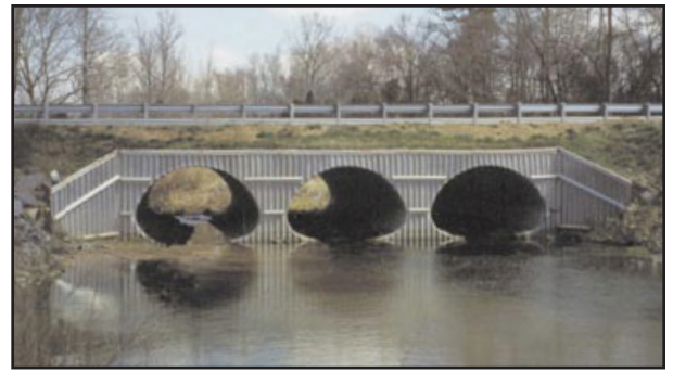
Aluminum Structural Plate - triple span stream crossing
