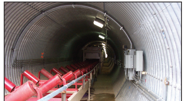
MULTI-PLATE® - 12' diameter reclamation tunnel
