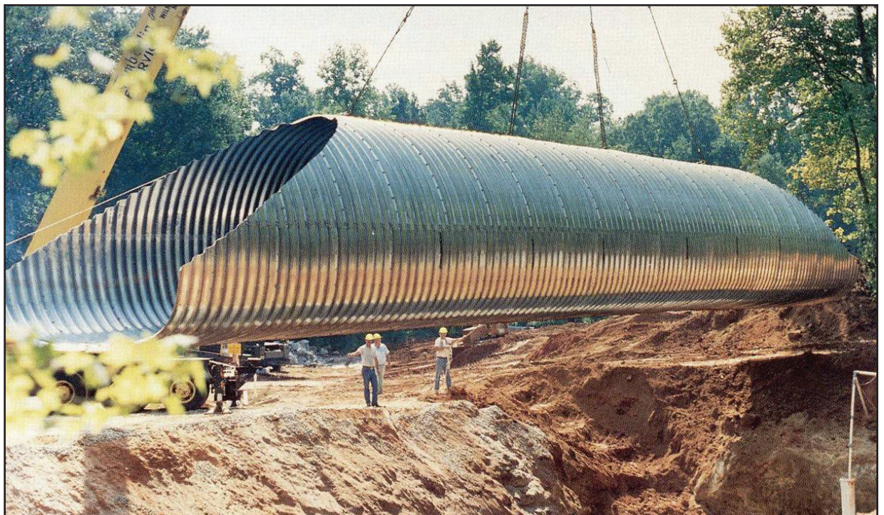
Aluminum Structural Plate - installation
