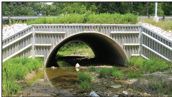
Aluminum Structural Plate - stream crossing
