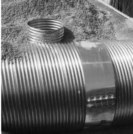
Some jobs may require special bands, such as rod and lug connection, flat bands, or dimple bands.
