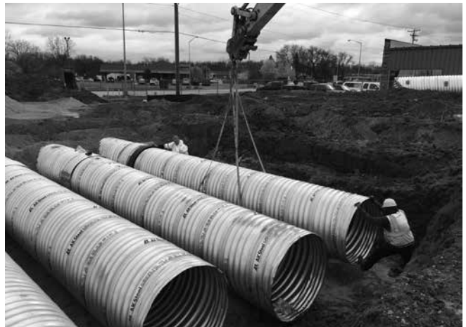
Lifting ALT2 CMP with nylon slings.
