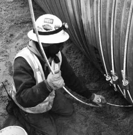
Some jobs may require special bands, such as rod and lug connection, flat bands, or dimple bands.
