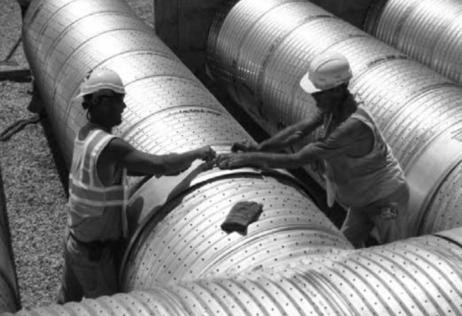
Installing a Hugger band on a perforated pipe.
