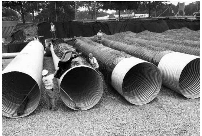
For large diameter pipes, the liner is shipped in rolls that are folded in half. The liner is rolled out over the crown of the pipe, unfolded, and covered over the pipe from the eight and four o'clock positions.
