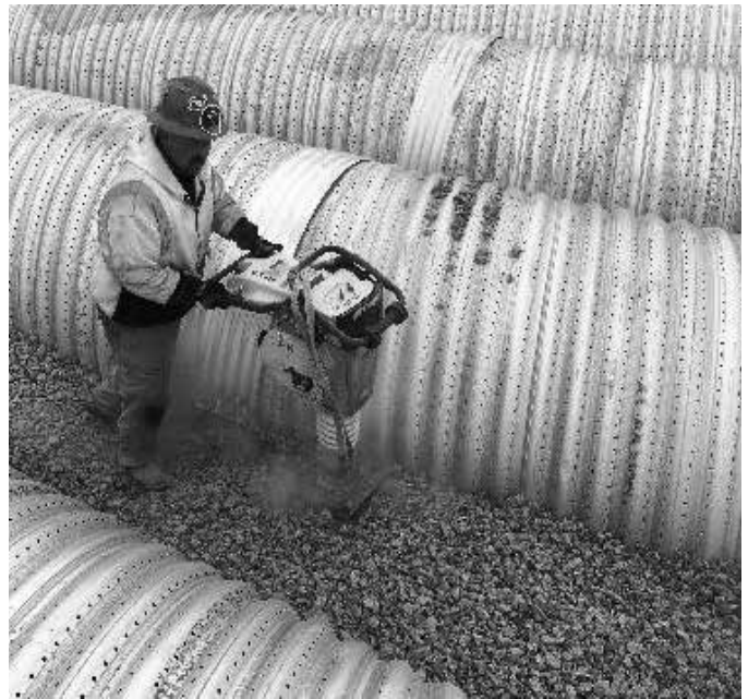
Compaction with vibratory equipment.
