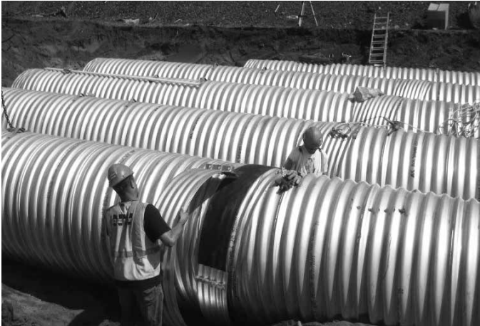
Tightening bolts on a corrugated band.
