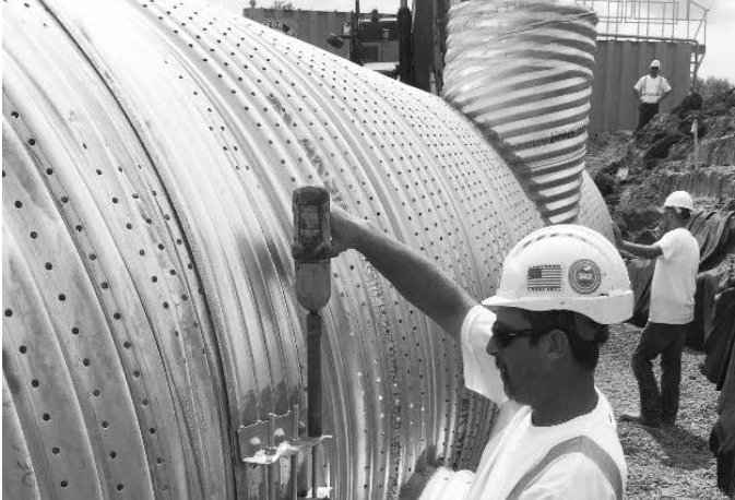
Tightening bolts on a corrugated band.
