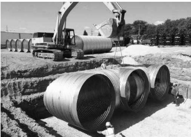
Lowering the header pipe section into place first.
