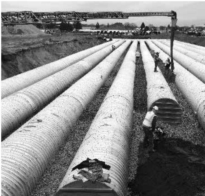
Placing backfill with a conveyor.
