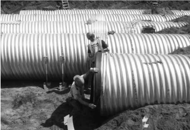
Installation of band with flat neoprene gasket.
