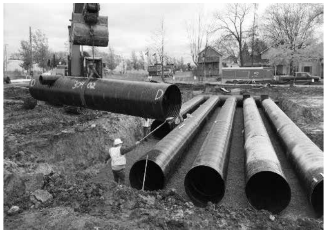
Lifting polymer-coated CMP into place with nylon slings.
