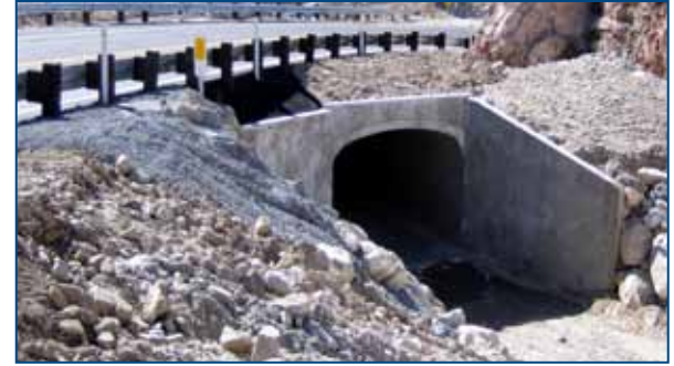
SR 18 (CA) – Caltrans emergency culvert replacement beneath popular state route (CON/SPAN)
