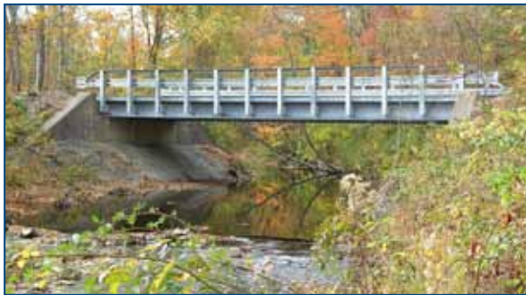
Pomfrey Road (CT) – rapid design-build solution for bridge replacement (U.S. Bridge)
