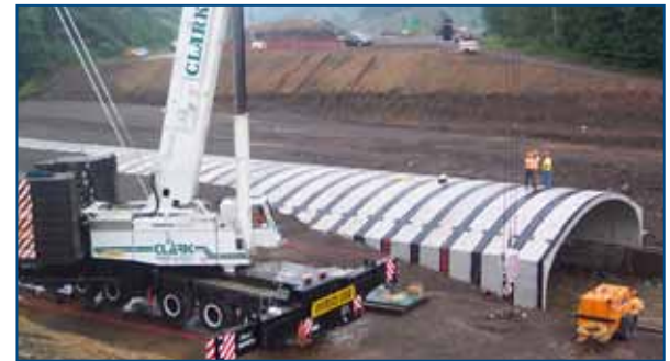
Interstate 88 (NY) – emergency replacement for DOT when storms washed out highway (CON/SPAN)
