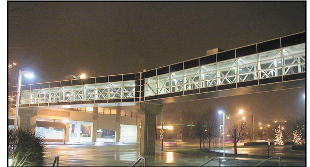
Box Truss - skywalk
