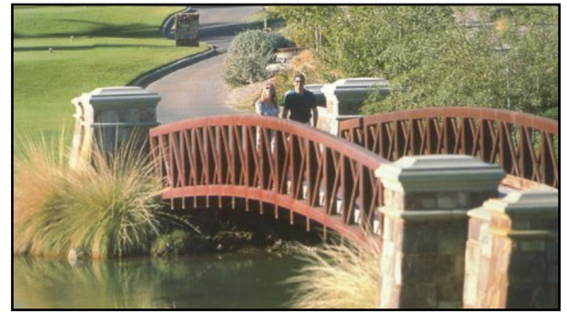
Pony Truss - golf course
