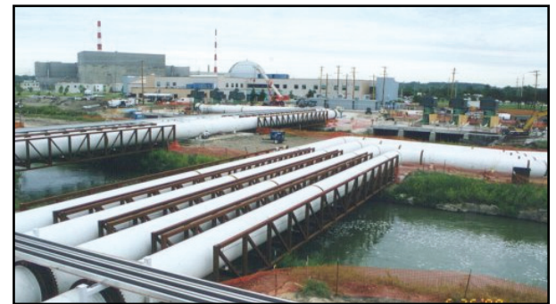
Connector™ Truss - utility crossing
