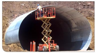
Mining Applications – plate structures have been utilized to extend and improve mine entrances, providing protection from falling rocks and debris. MULTI-PLATE structures are widely used for aggregate tunnels and utility conduit.
