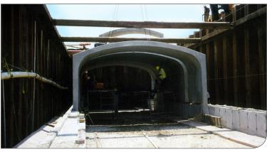
**Discharge Structures** – durable precast structures transport pumped waters and provide protection during harsh weather conditions
