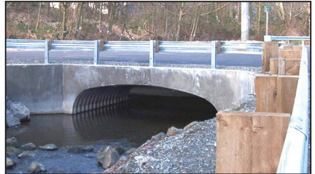
Aluminum Box Culvert - stream crossing
