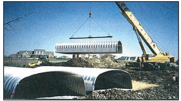
Aluminum Box Culvert - multi-cell installation
