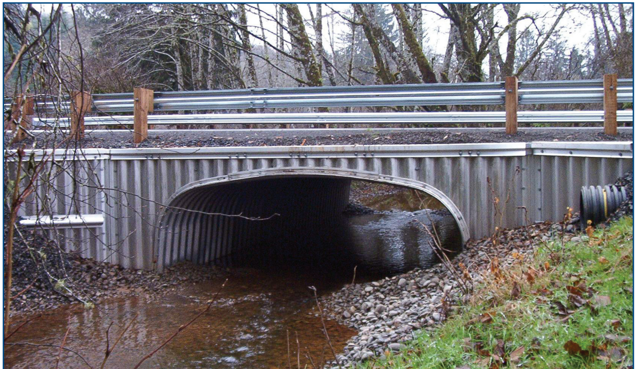
Aluminum Box Culvert - relining - stream crossing
