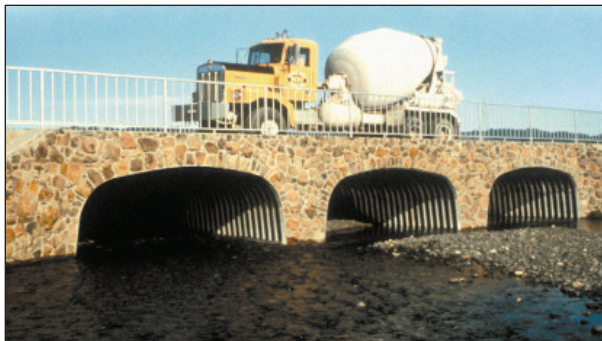
Aluminum Box Culvert - county road bridge
