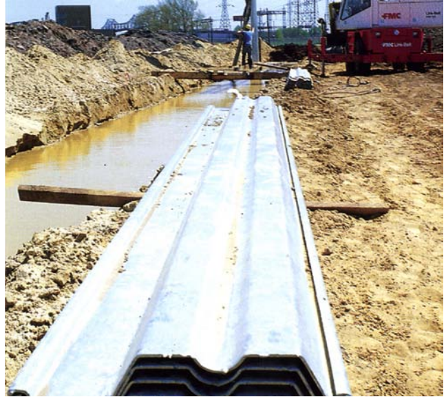
The nestability of Contech Metric Sheeting facilitates shipping and handling.
