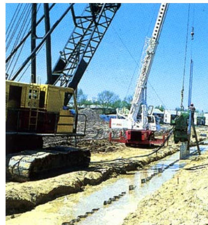
Contech Metric Sheeting offers a tight, metal-to-metal interlock on this cut-off wall under a dike.
