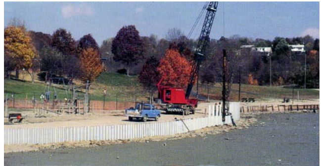
Contech Metric Sheeting, fabricated from ALUMINIZED STEEL Type 2 for added corrosion resistance, will check erosion along this lake shore in a county park.
