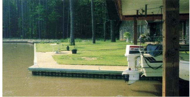
Relative low-cost, attractive appearance and proven durability of medium-weight Contech Metric Sheeting have made it a popular choice for waterfront installations like this.
