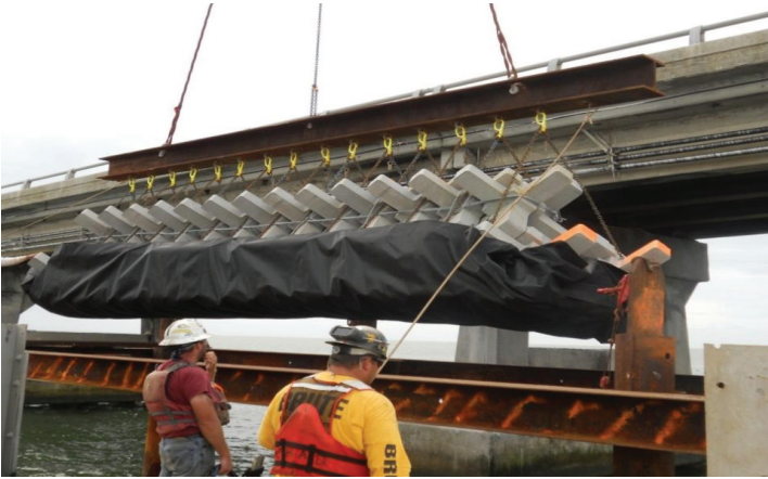
Herbert C. Bonner Bridge - NC12 - NCDOT Outer Banks, North Carolina
