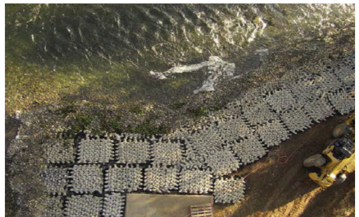
Tuolumne River Bridge - Caltrans Hickman, California
