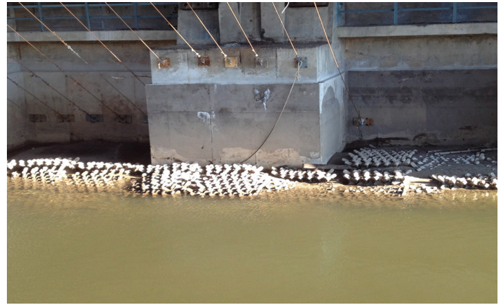
Route 35 Cheesquake Creek Bridge - NJDOT Morgan, New Jersey
