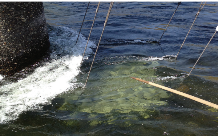
US95 Spalding Bridge - ITD Lewiston, Idaho
