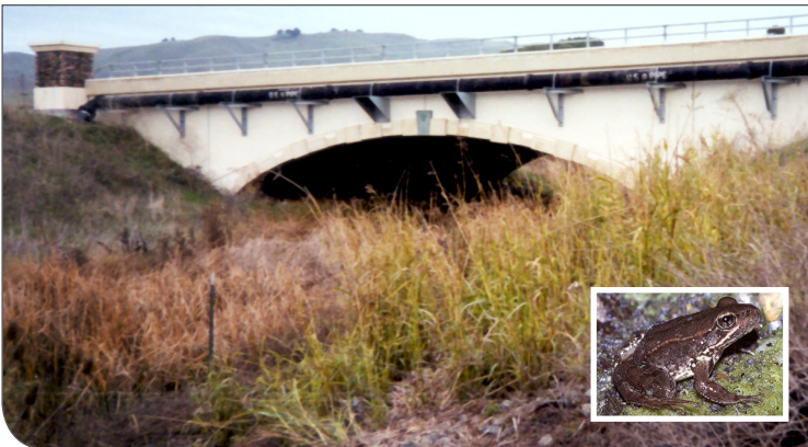
California Red-Legged Frog – strict environmental permitting called for a bottomless arch that protects this endangered frog
