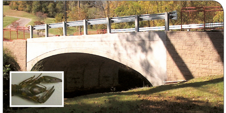
Nashville Crayfish – roadway crossing uses a bottomless precast arch to ensure protection of the Nashville Crayfish
