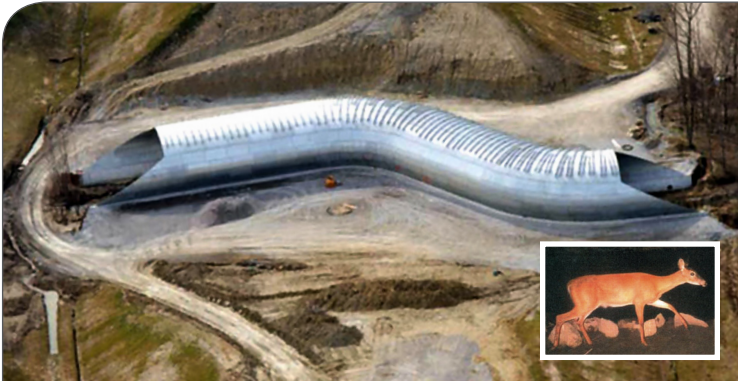
Deer Crossing – this animal crossing allows deer to pass safely beneath a busy highway
