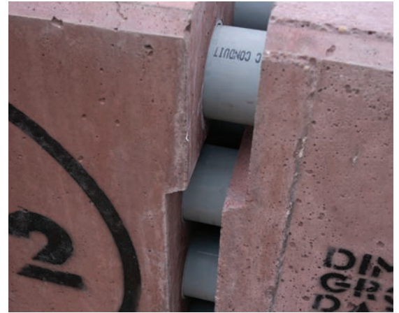
- Shear key & joint system
